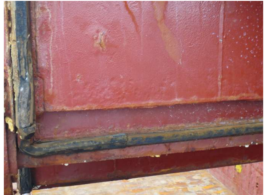
Poor rubber packing.
